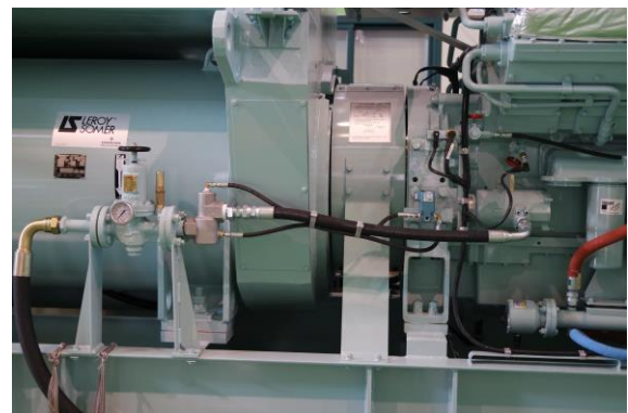
<Compressed Air Starter>
