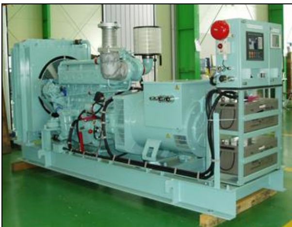
Emergency Generator Set (150kW, 60Hz)
