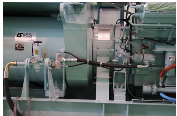
<Compressed Air Starter>
